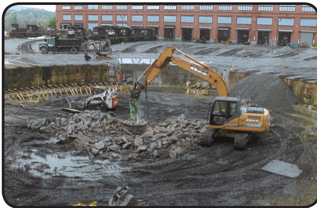
Digging out the old pivot point and installing the new circle track
