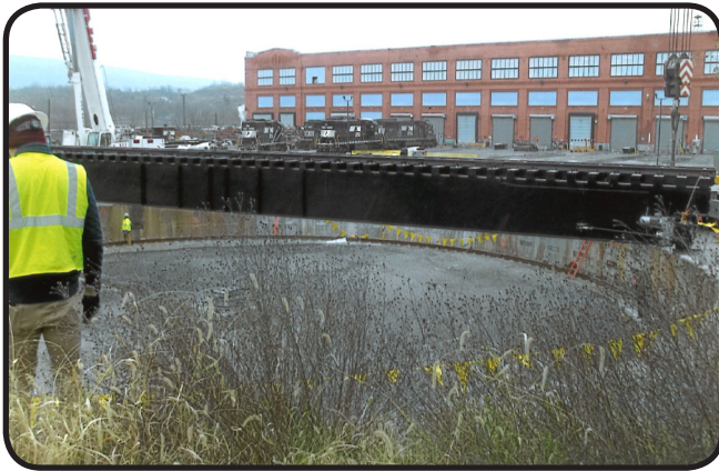
Getting lined up on the pit to begin the lowering process
