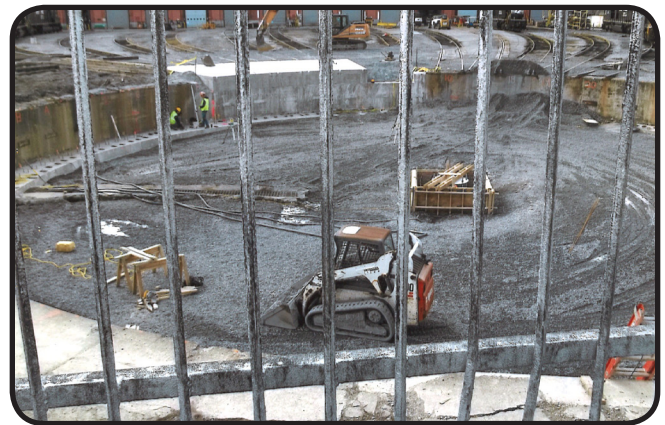
Pouring the new pivot point and finishing grading the pit floor
