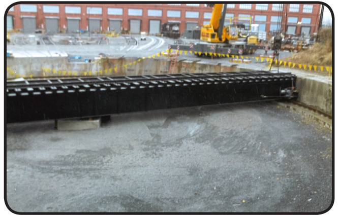
Lowered onto the pivot point and the edge tracks
